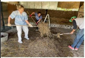
They learned two ancient techniques that our ancestors used for building walls. Pajarcilla uses cut up straw, then adds mud with a high clay content and water. This gets mixed up well. The other kind is called Cob: Once again they use mud with a high clay content and they make sort of a dough. The straw has to be very well cut up. These two items have to be integrated well. Although they got dirty,
